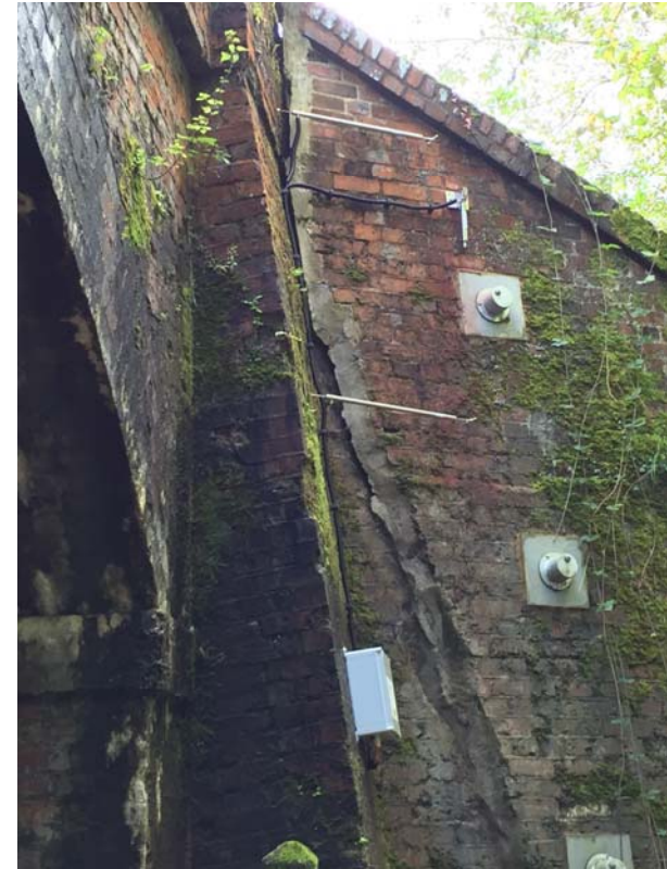
Critical Structure Monitoring
