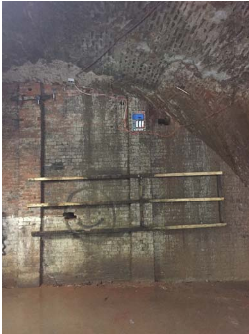
Critical Structure Monitoring
