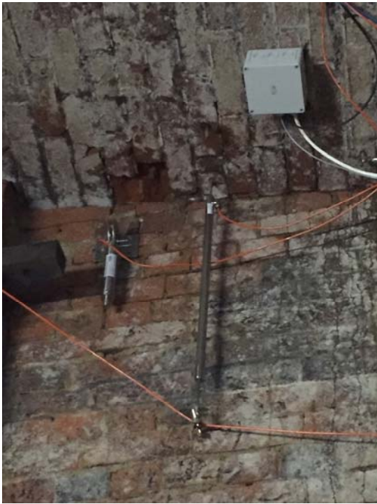
Critical Structure Monitoring
